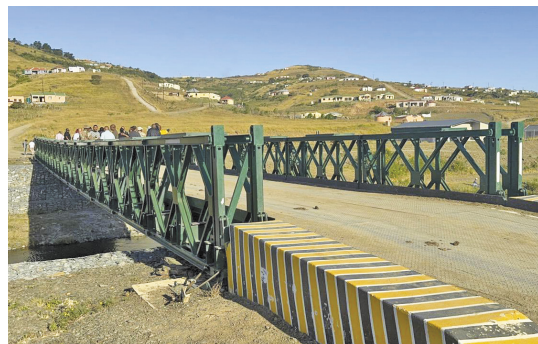
SA Army Engineers are building sturdy steel structures as part of the Welisizwe Bridges Programme.
