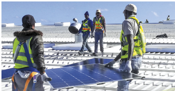
Solar panels being installed at Dairy Group SA
