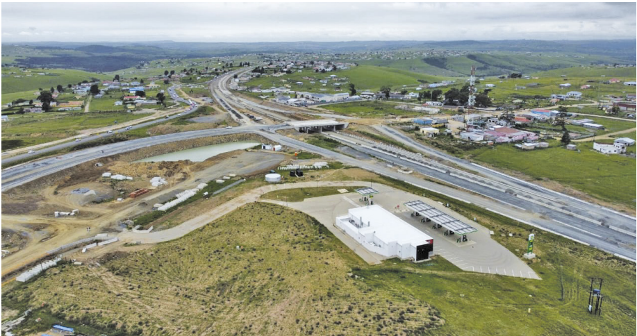
The new Ndabakazi Interchange on the N2 in the Mnquma Local Municipality near Gcuwa (Butterworth) greatly enhances the safety of users.
