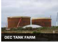
OEC TANK FARM
