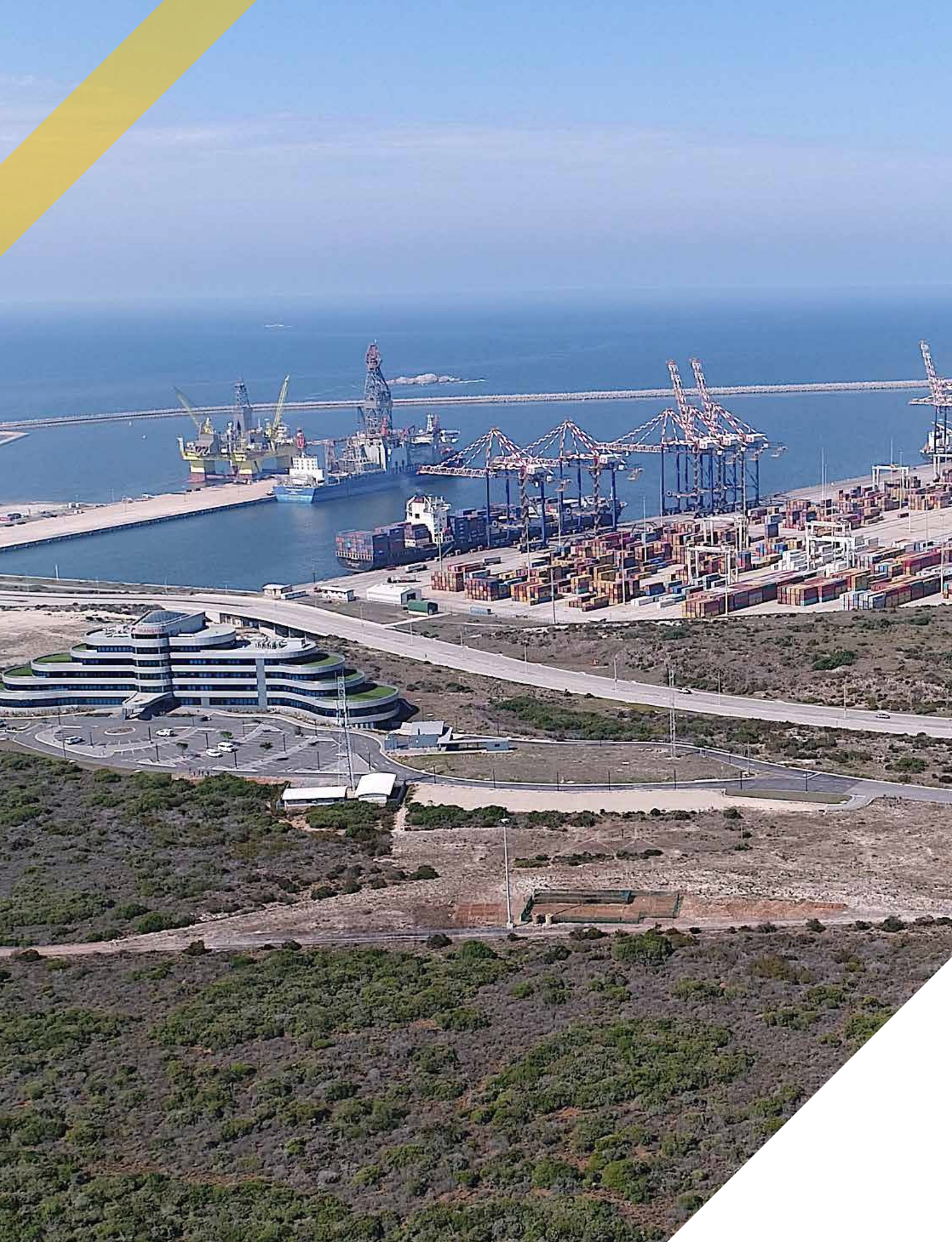
Deepwater Port of Ngqura, strategically situated within the Coega SEZ Complex, Zone 1.
