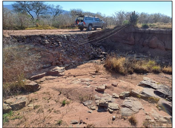
Plate 5 (Left): drainage line on the downriver side of the stream crossing near TP7. Note Alluvial banks underlain by sedimentary rock. Plate 6 (Right): Existing stream crossing/culvert at TP7 with undermining at the abutments – Note poor drainage of the upriver section through the bridge fill material.
